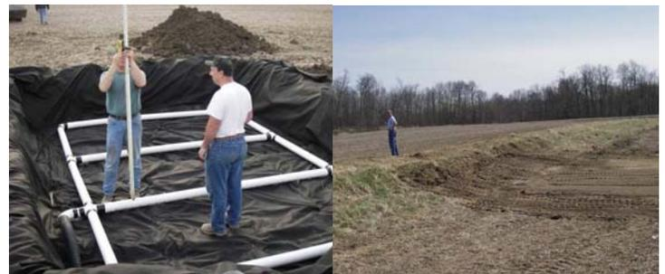
A blind tile inlet installation prior to the placement of gravel (left) and the completed practice (right). Photos from USDA-ARS.
